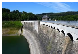
c) Dam and bridge
