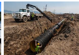
d) Poor soil drainage
