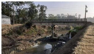
b) River excavation
